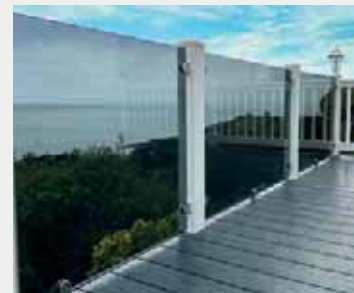
Fixed with stainless steel glass clamps
